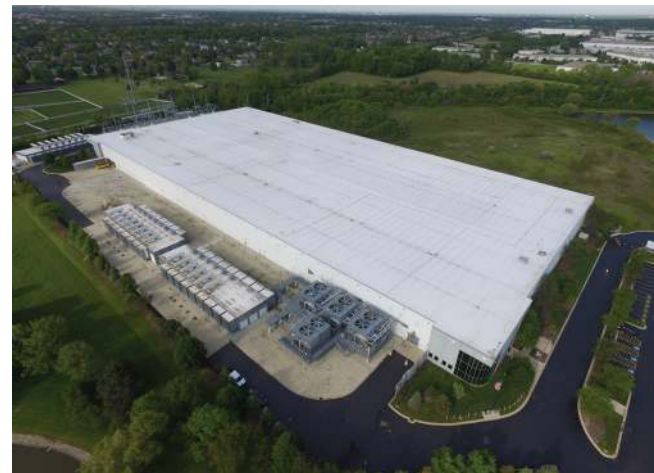
Chicago – Aurora I Data Center
